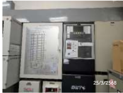
Fire Alarm Control Panel
